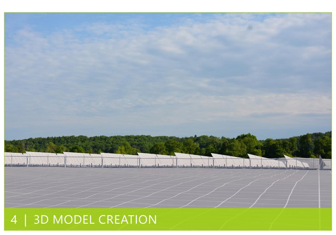
3D models of the Facility are built based on specifications of the PV panels, racking, fencing, and other components for each of the PV panel configurations and set back scenarios. These models are then placed in the correct geographic position within the 3D model.
